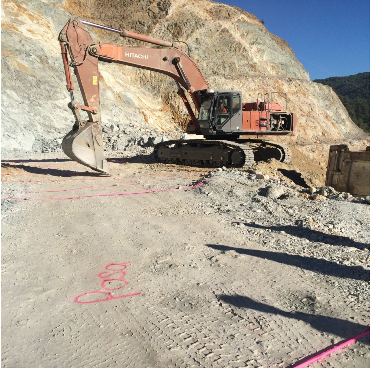
Figure 3.10.3.1: Çukuralan Bench Face and Grade Control
